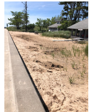
Sink holes on properties along north channel pier.
