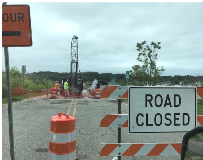
Drilling pilot holes for new road construction
